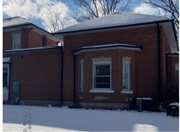
Plate 44: Detail of east elevation bay window
