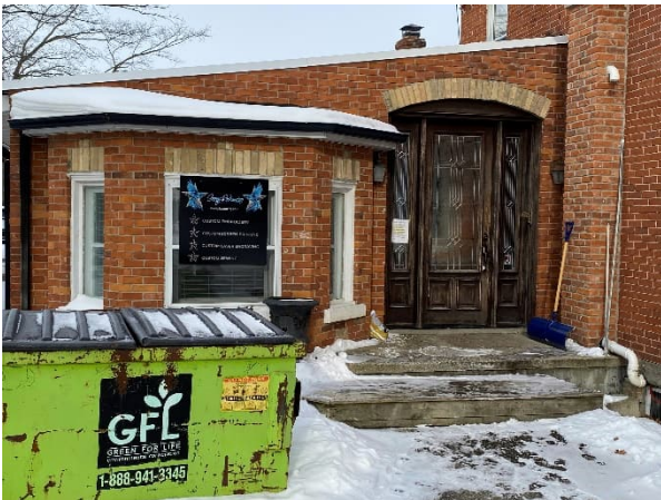
Plate 45: South entrance to side addition
