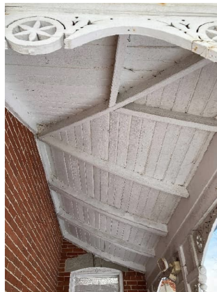
Plate 31: Bellcast roof of the side porch
