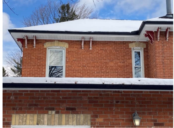
Plate 37: Upper storey windows of main block west elevation showing possible later replacements of some decorative element such as brick arch heads
