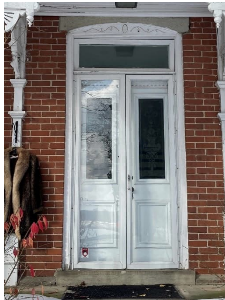
Plate 27: Main entrance doorway (south elevation)
