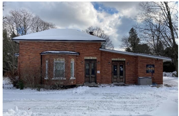
Plate 42: North elevation of rear/side addition
