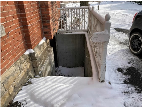
Plate 38: Basement access on west elevation
