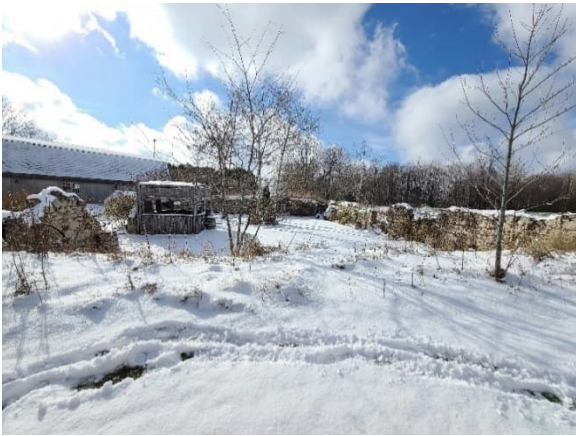
Plate 14: Barn foundation ruins, looking southwest
