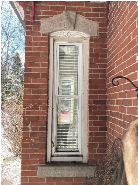
Plate 26: Detail of box bay side windows
