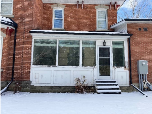
Plate 36: Enclosed porch of east elevation
