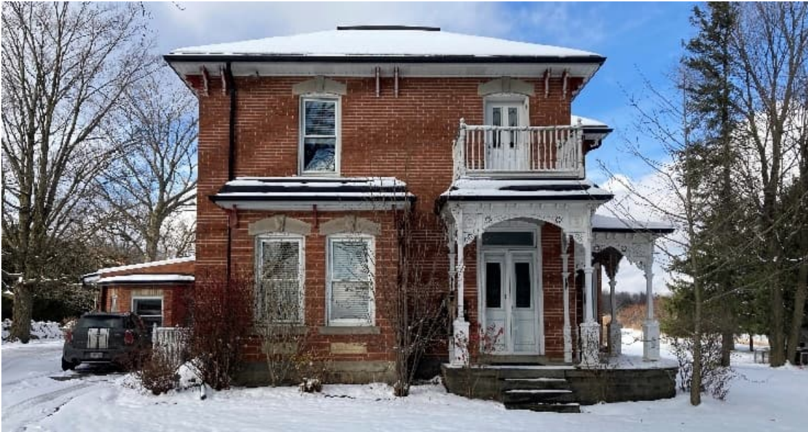
Plate 16: South (front) elevation, facing Charleston Sideroad
