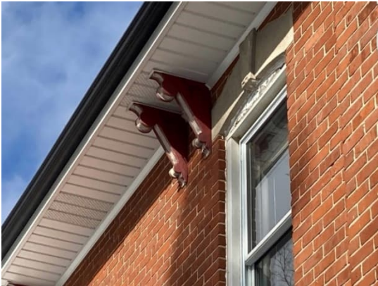
Plate 22: Overhanging eaves and paired bracket detail
