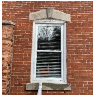
Plate 23: Main block window example
